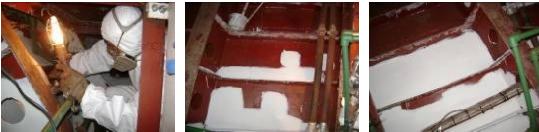
4. Final coat fwd water tank*
