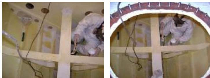
4. Final coat fwd water tank*
